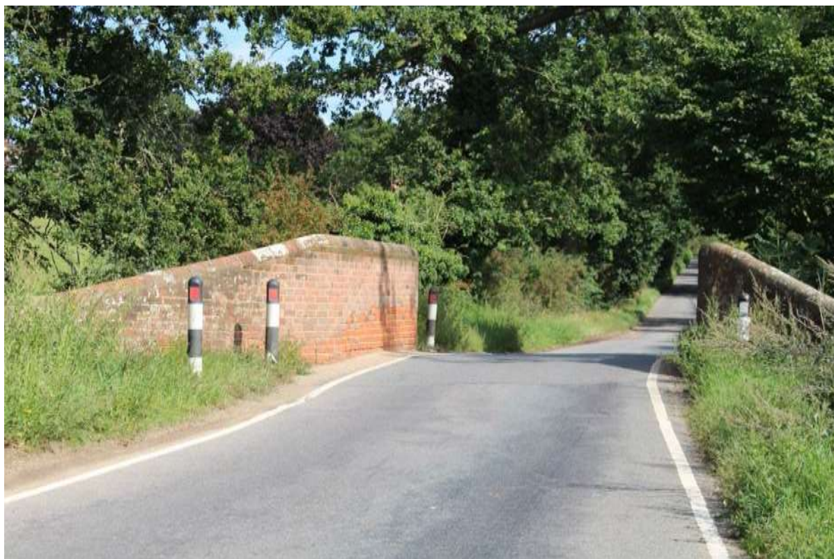
Boot Street bridge
