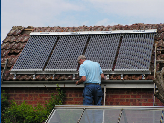
Solar Water - generates hot water
