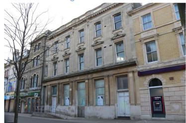
of stonework and reconfigure the ground floor windows to restore the entrance to the central bay of the building, as per the original design of the building. This will incorporate repositioning the existing ramp which would greatly improve the appearance of the building.
